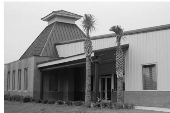
The new SWUCI Field Maintenance Facility
