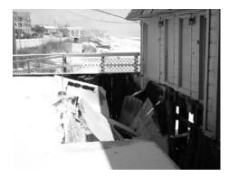
Beach erosion has been a problem for beach front homes. Hurricane Ivan destroyed the retaining wall and the additional surge of Hurricane Dennis washed away the remaining sand. Without the support of the retaining wall, the parking lot collapsed.
