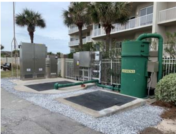
Lift Station rehabilitation
